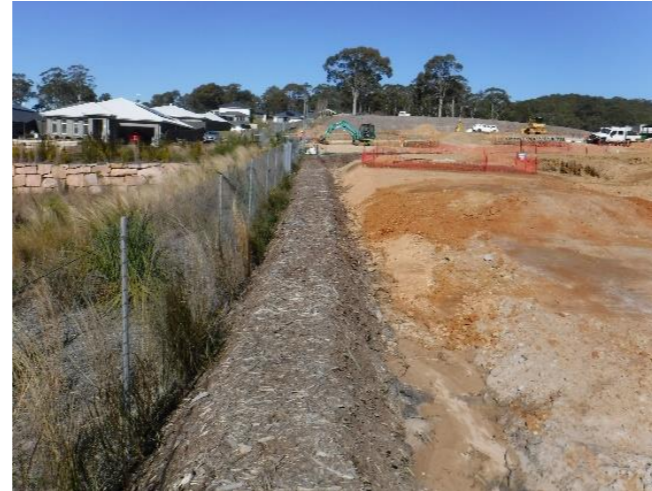
Example photo of a compacted mulch berm on low grades.
