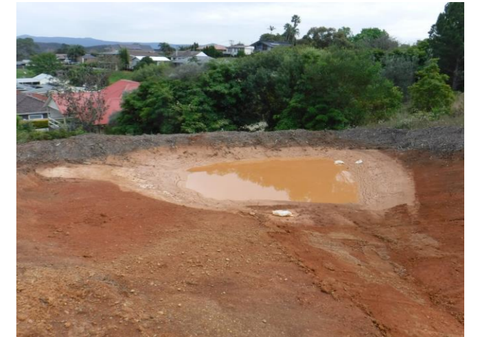
Example photo of an excavated sediment trap with mulch filter berm.
